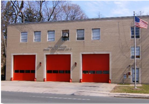
Station 11 - 150 Sisson Ave Parkville / West End Engine 11: 3,551 Ladder 5: 2,284 Total 2018 Calls: 5,835
