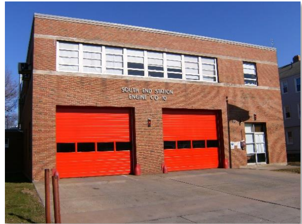
Station 10 - 510 Franklin Ave South End / South Meadows Engine 10 Total 2018 Calls: 2,815
